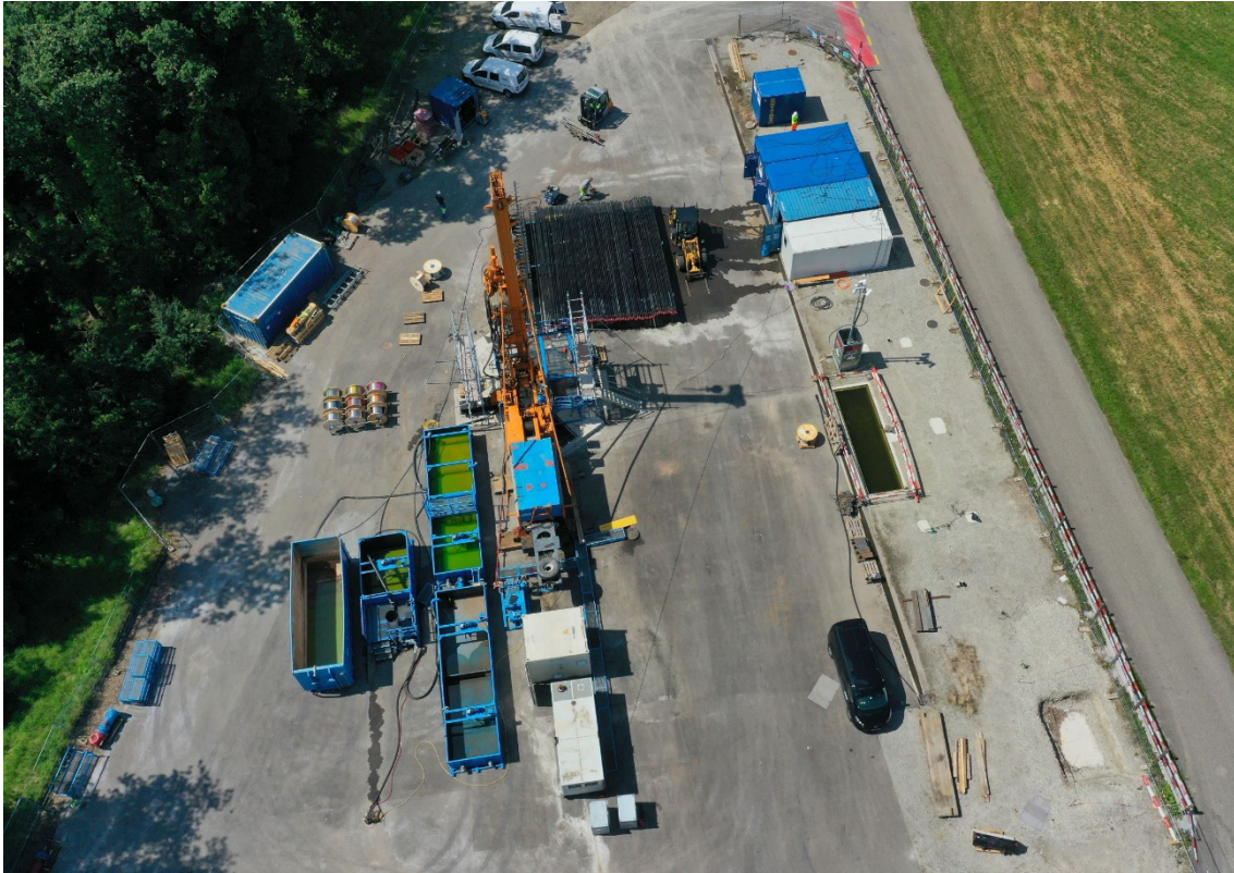
Fig. 3-1: Aerial view of the drill site during installation of the MPS
