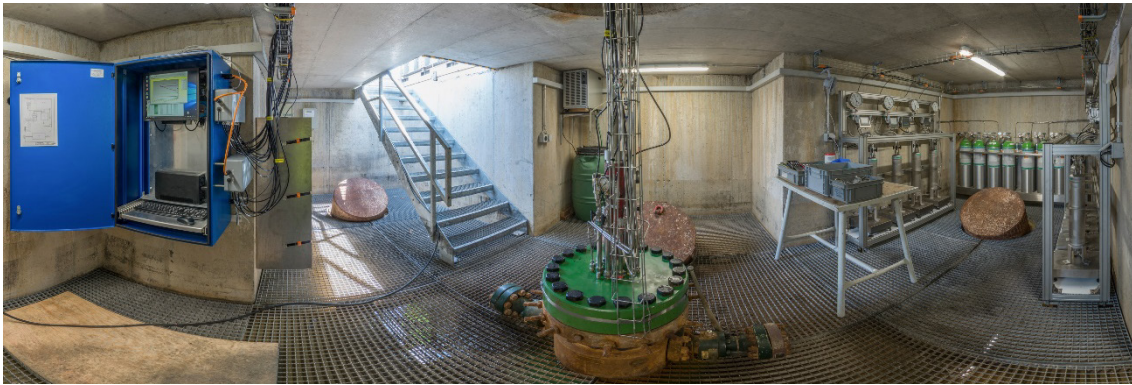
Fig. 4-1: Panoramic view of the borehole cellar with (from left to right) the DAS, entrance, wellhead with inflate and monitoring lines and the pressure control system with pressure vessels and gas bottles
