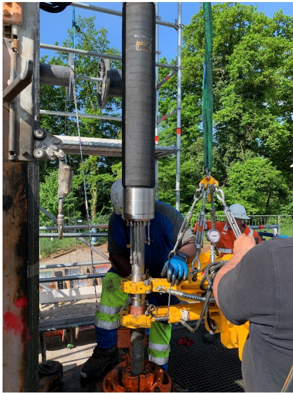
Fig. 2-2: Installation of a packer element on the central tubing
