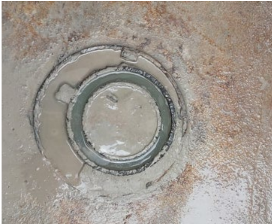
Fig. 3-16: Borehole BAC1-1 completely backfilled and casing extensions cut
