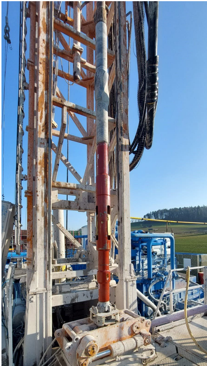
Fig. 3-15: 11" underreamer before RIH
