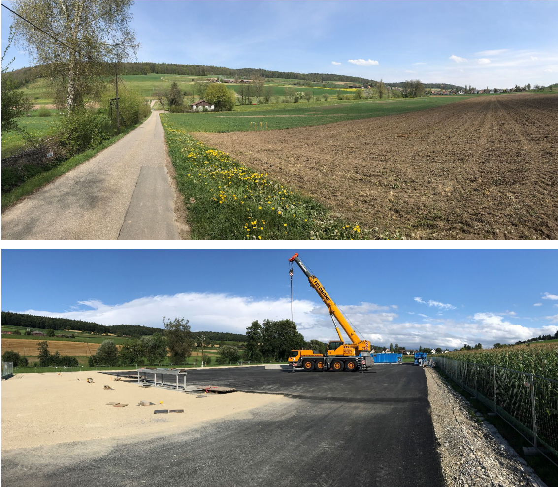
Fig. 3-1: Drill site before (top) and after (bottom) construction
