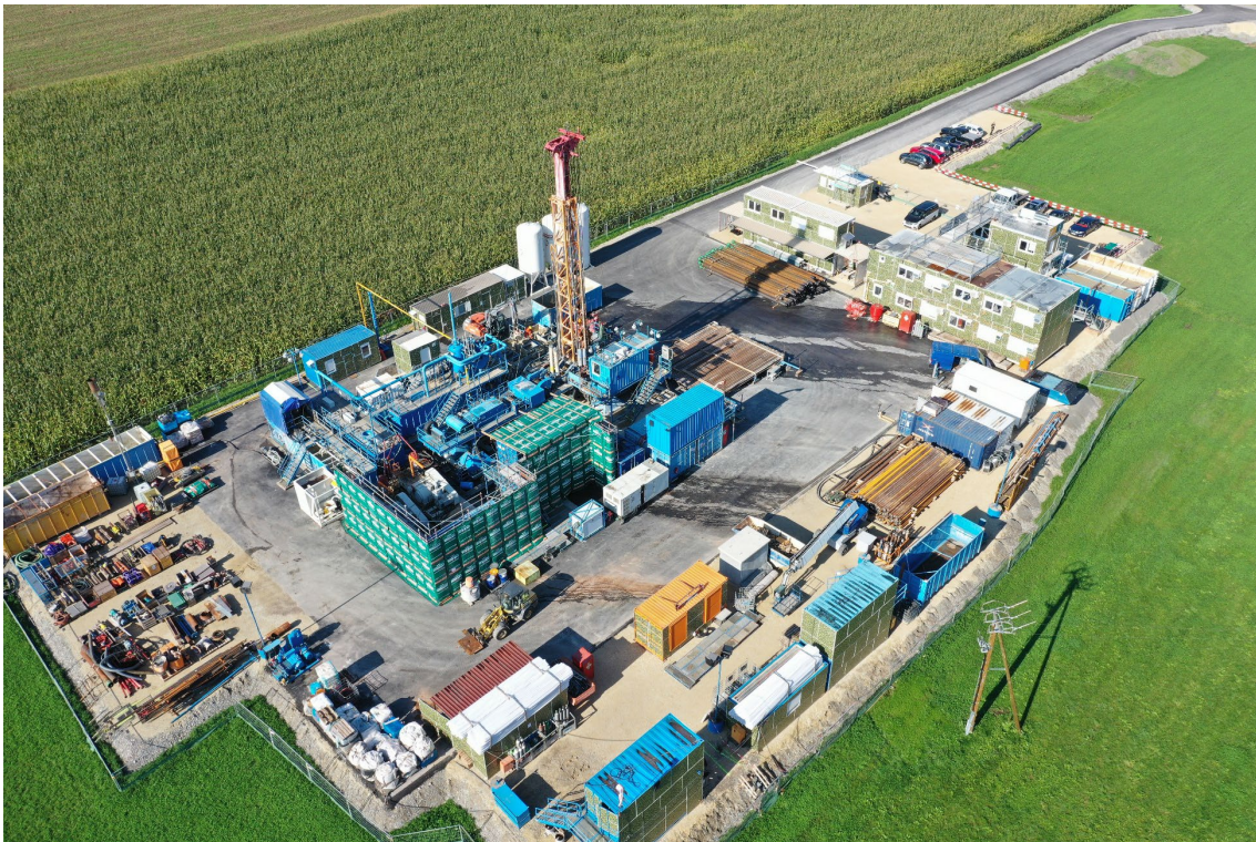
Fig. 3-2: Drill site after installation of the drilling rig and peripheral facilities
