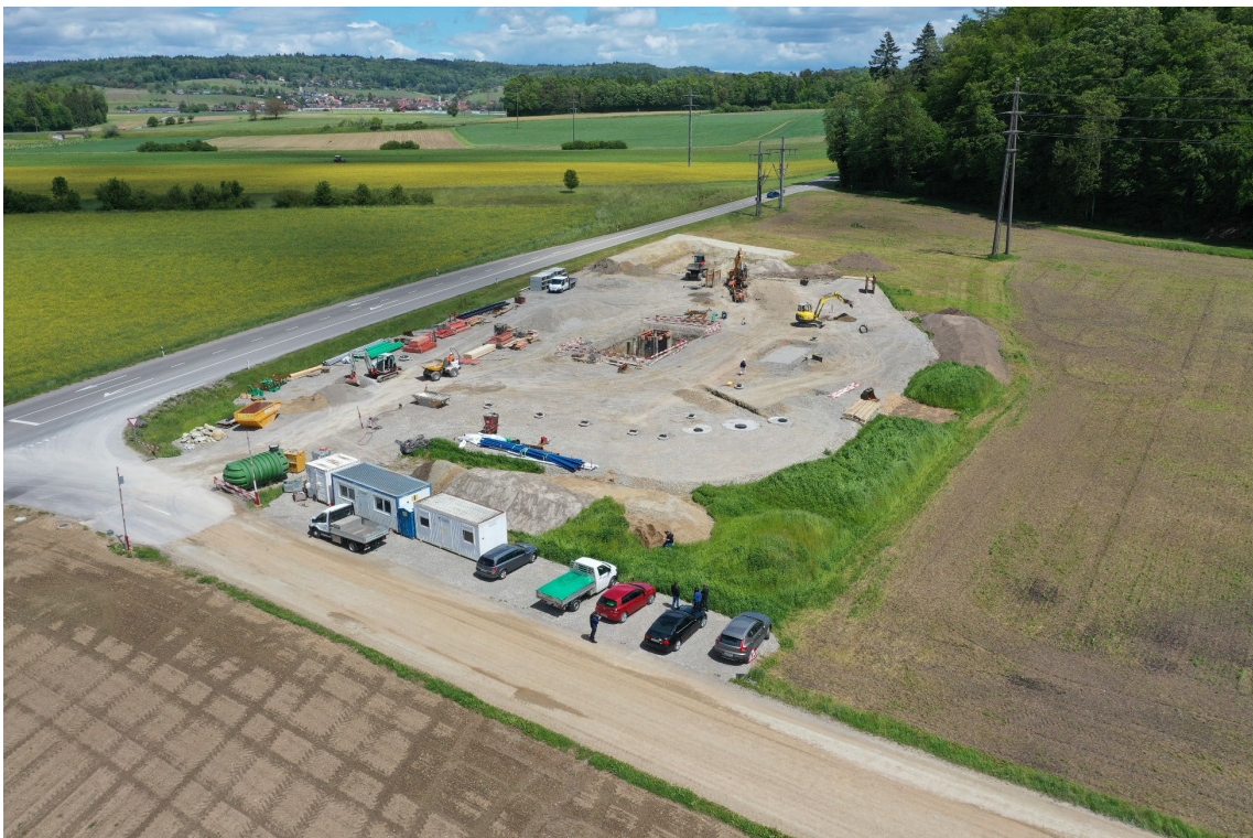
Fig. E-4: Construction of well cellar
