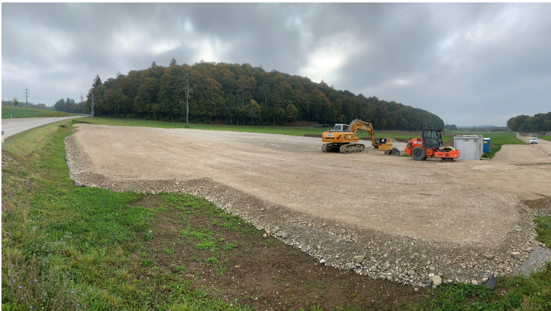
Fig. E-3: Gravel layer on soil
