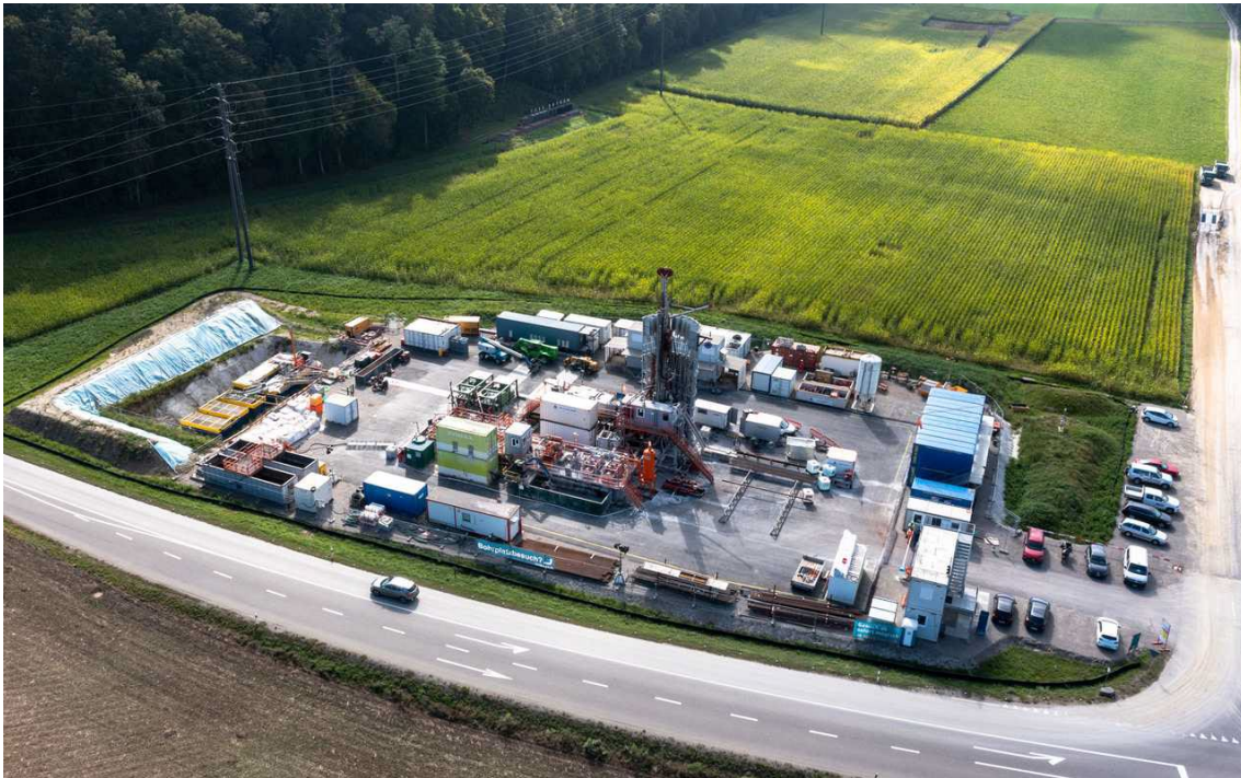
Fig. 3-1: Picture of the drill site
