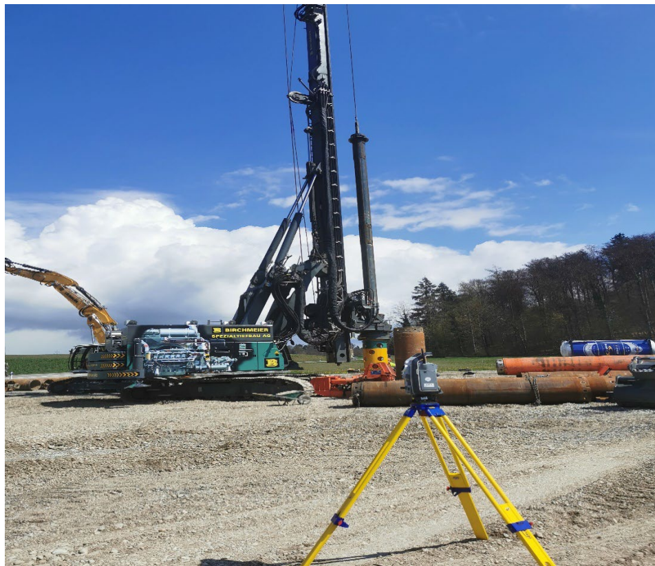
Fig. 3-2: Drilling the hole for the 13 \frac{3}{8} " standpipe
