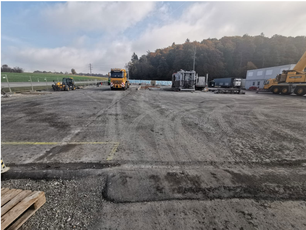
Fig. E-5: Paving the site
