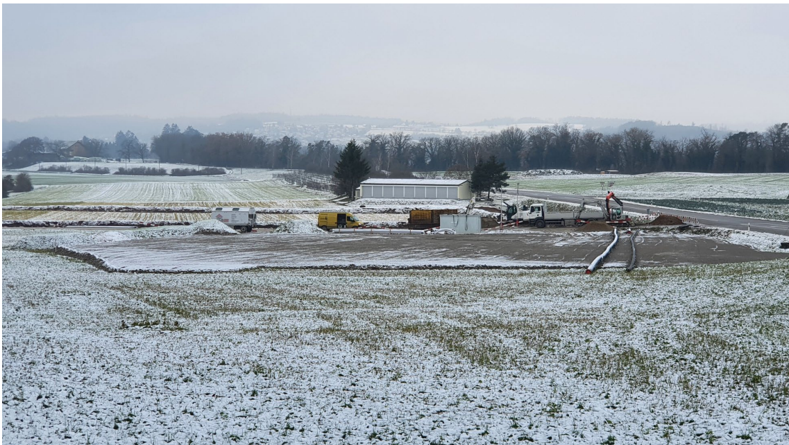
Fig. E-2: Trench excavation (above) and piping (below)
