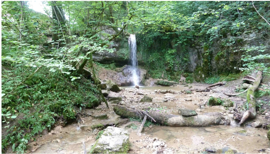
Fig. 24: Knickpoint in LP-5 (northwest of Linn, 490 m a.s.l.), interpreted as lithologically controlled by higher substrate resistance within the Villigen-Formation (LP-5).
