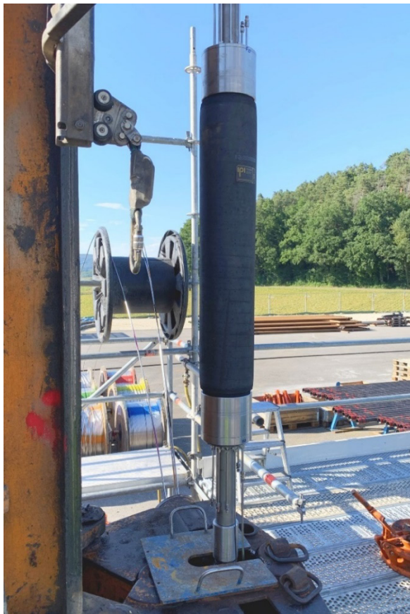
Fig. 2-3: Installation of a packer element on the central tubing
