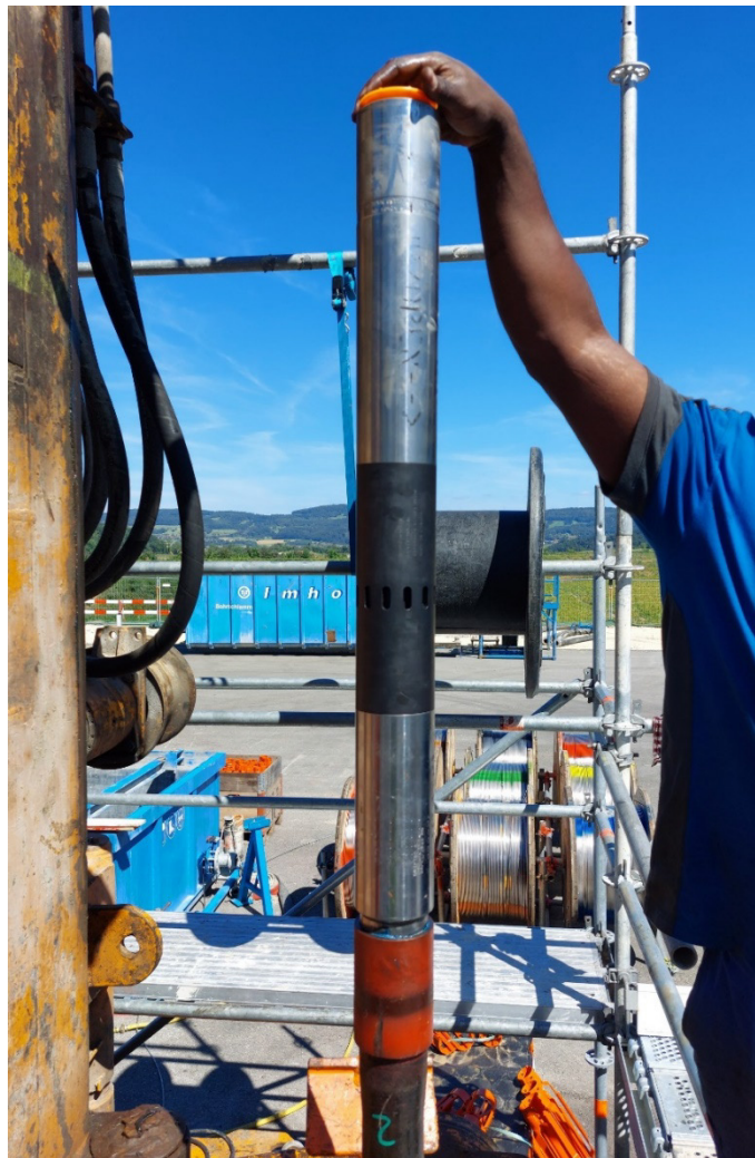
Fig. 2-6: Installation of a sliding sleeve on the central tubing
