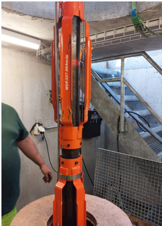
Fig. 2-2: Two centralisers were used to help guide the lowermost section of the MPS
