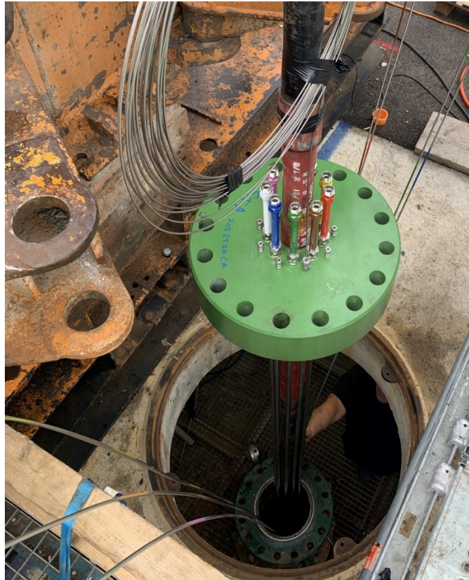
Fig. 2-9: Lowering of the landing spool with fittings for standpipes and packer inflate lines
