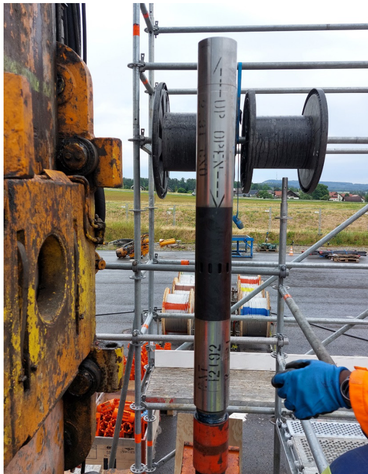
Fig. 2-5: Installation of a sliding sleeve on the central tubing
