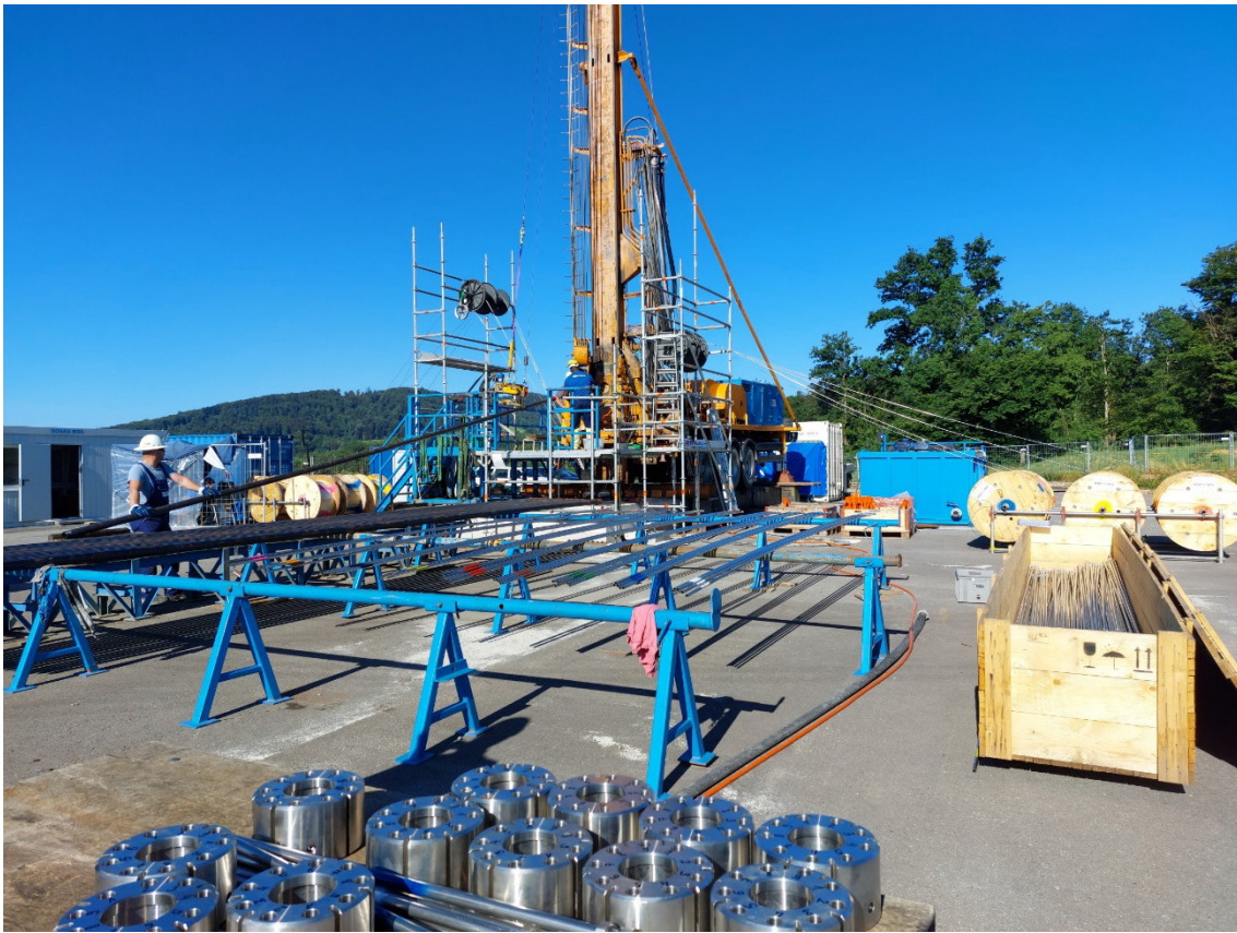
Fig. 3-1: Setup of the workover rig during installation of the MPS
