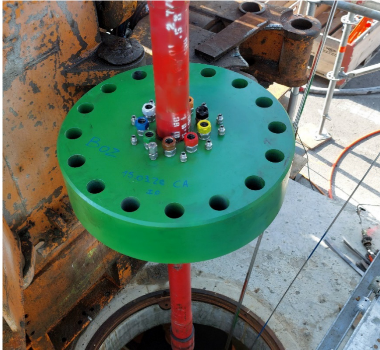
Fig. 2-8: Lowering of the landing spool with fittings for standpipes and packer inflate lines
