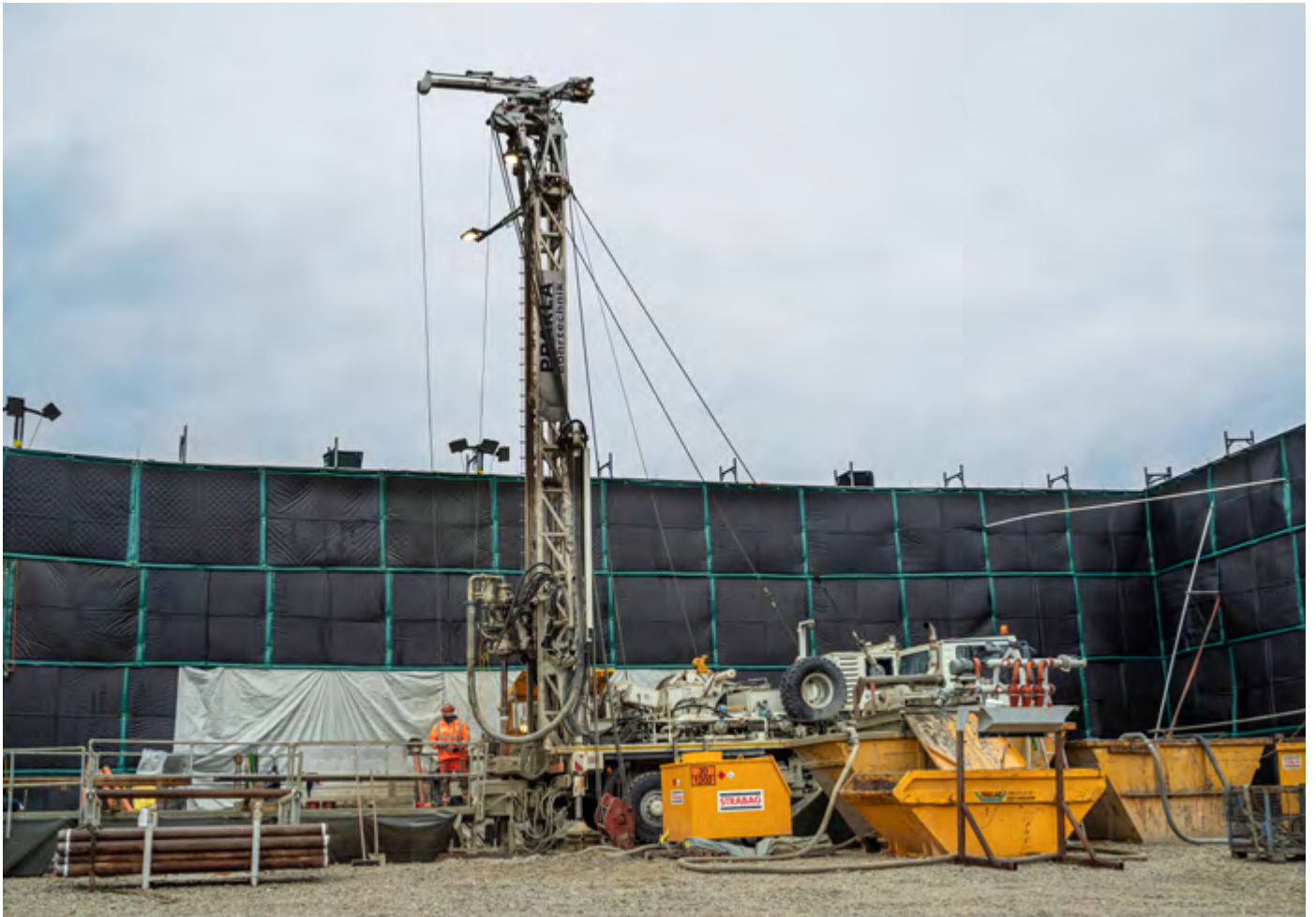
Above: The drill site of the Adlikon-Dätwil Quaternary borehole with the drilling rig. The wall protects the adjacent houses from noise. Below: The drilling crew pulls a drill core to the surface. At this point, it is still attached to a cable in the borehole.
