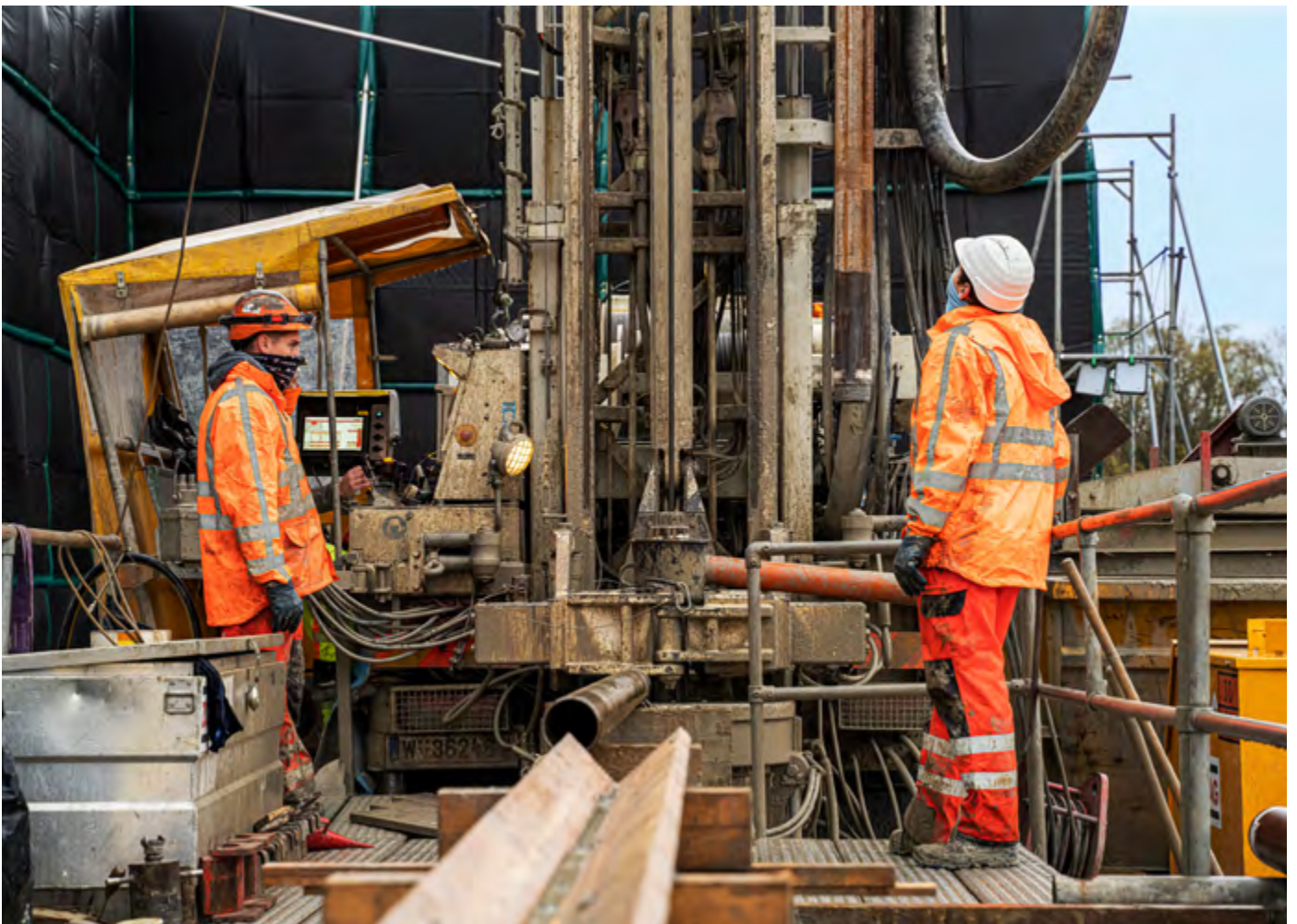
Above: The drill site of the Adlikon-Dätwil Quaternary borehole with the drilling rig. The wall protects the adjacent houses from noise. Below: The drilling crew pulls a drill core to the surface. At this point, it is still attached to a cable in the borehole.
